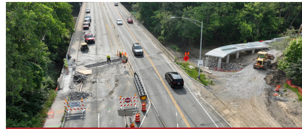
West North Broadway Over Olentangy River In Progress
