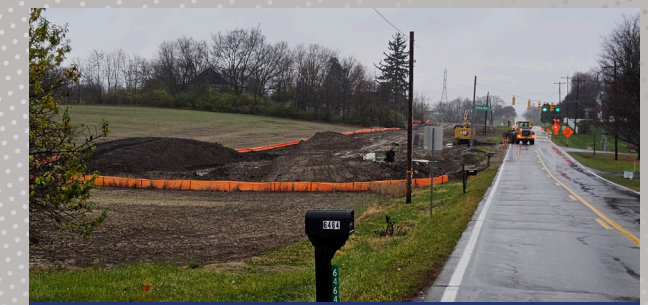
Kropp Road Drainage Outlet Part 1
