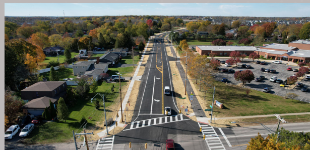
Renner Road (Alton & Darby Creek Road to Spindler Road)
