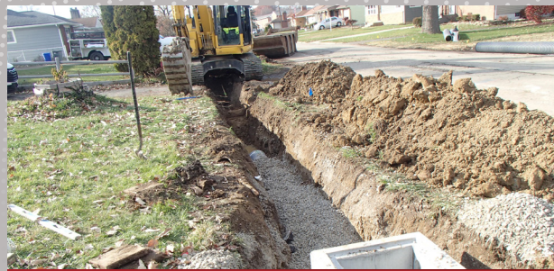
Case Road Area Storm Sewer Replacement
