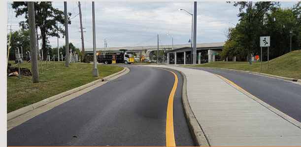
2025 County Resurfacing Program
