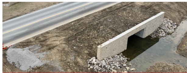
Eiterman Road Over South Fork Indian Run In Progress
