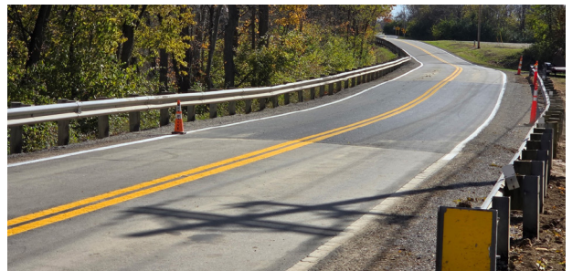
Pontius Road Over Tributary of Little Walnut Creek
