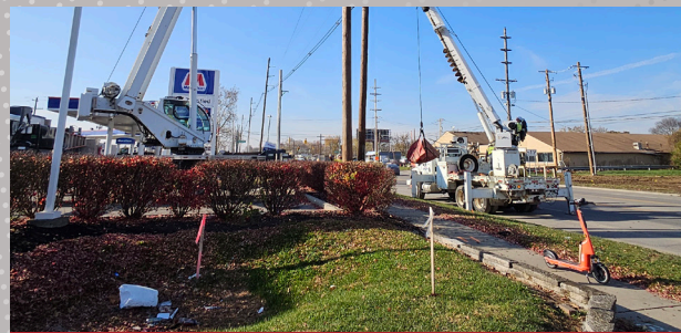
Frank Road at Brown Road / Hardy Parkway Street MELP Relocation
