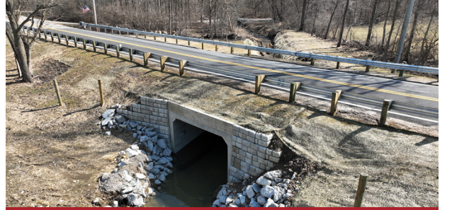
Roberts Road Over Morris Ditch
