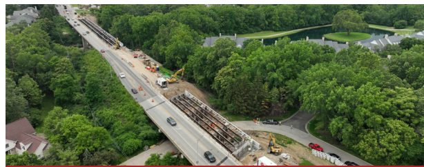
Trabue Road (Lakeshore Drive to Riverside Drive) In Progress
