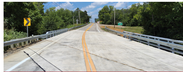
General Bridge Maintenance
